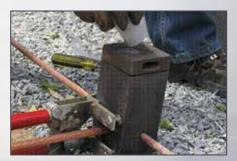
safety of the contained, high-temperature reaction; the irreversible connection; the lack of loosening or corrosion at the weld site; and no need for an outside power source.
